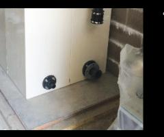
Alternatively, if the plinth tolerance cannot be achieved, the use of levelling steels will allow you to take up any irregularities with shims up to a maximum of 18mm.
