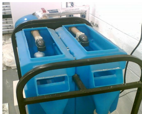
Internal back-up supply module with twin supplies and Type AB air gaps.
