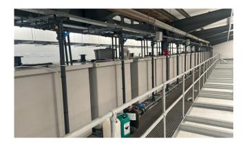
The project brief from J. Pao and Co. Ltd was both clear and uncompromising, reflecting the precision required for a food-grade facility. The company required 50 one-piece GRP cold water storage tanks, each manufactured to exact custom dimensions of 2000 x 1200 x 1100mm. These tanks needed to be fully WRAS-approved to ensure compliance with stringent hygiene regulations and constructed from corrosion-resistant materials suitable for long-term use in this demanding environment.
