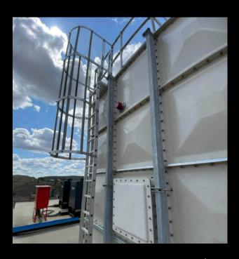
**TANK DIMENSIONS:** 8m x 7m x 4m deep (x2 installed; third planned for 2026)
